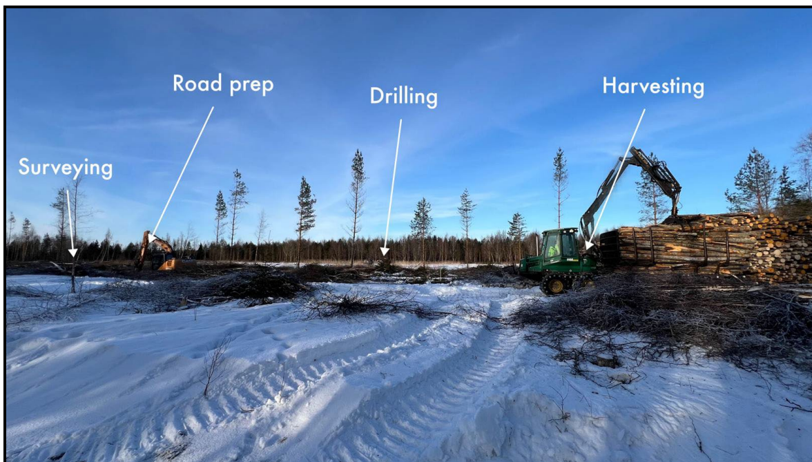
Korsnäs REE program involved use of regrowth tree crops for local community heating purposes.
